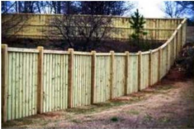
Figure 155.5302.F.1: Fence with finished side out.
